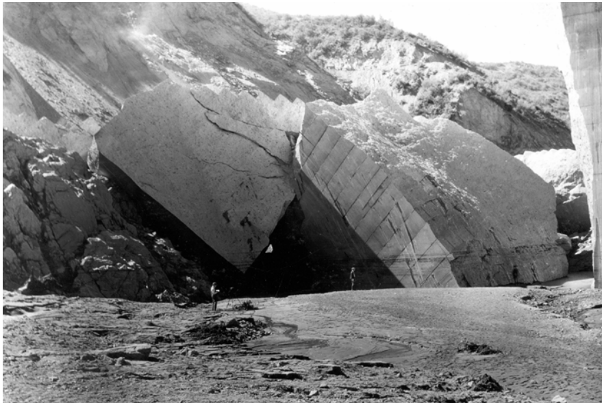
St. Francis Dam, Concrete Debris Blocks (Attribution: U.S. Geological Survey Photographic Library) Figure 5
