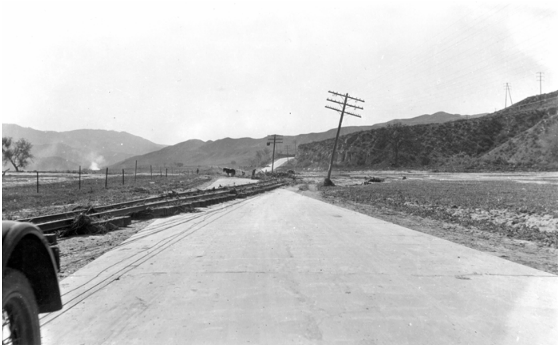
Dislocated railroad tracks (Attribution: U.S. Geological Survey Photographic Library) Figure 9
