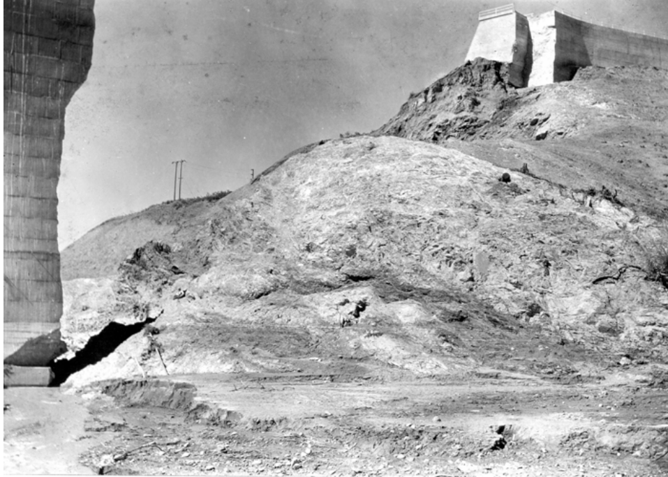
St. Francis Dam, Former West Abutment (Attribution: U.S. Geological Survey Photographic Library) Figure 6
